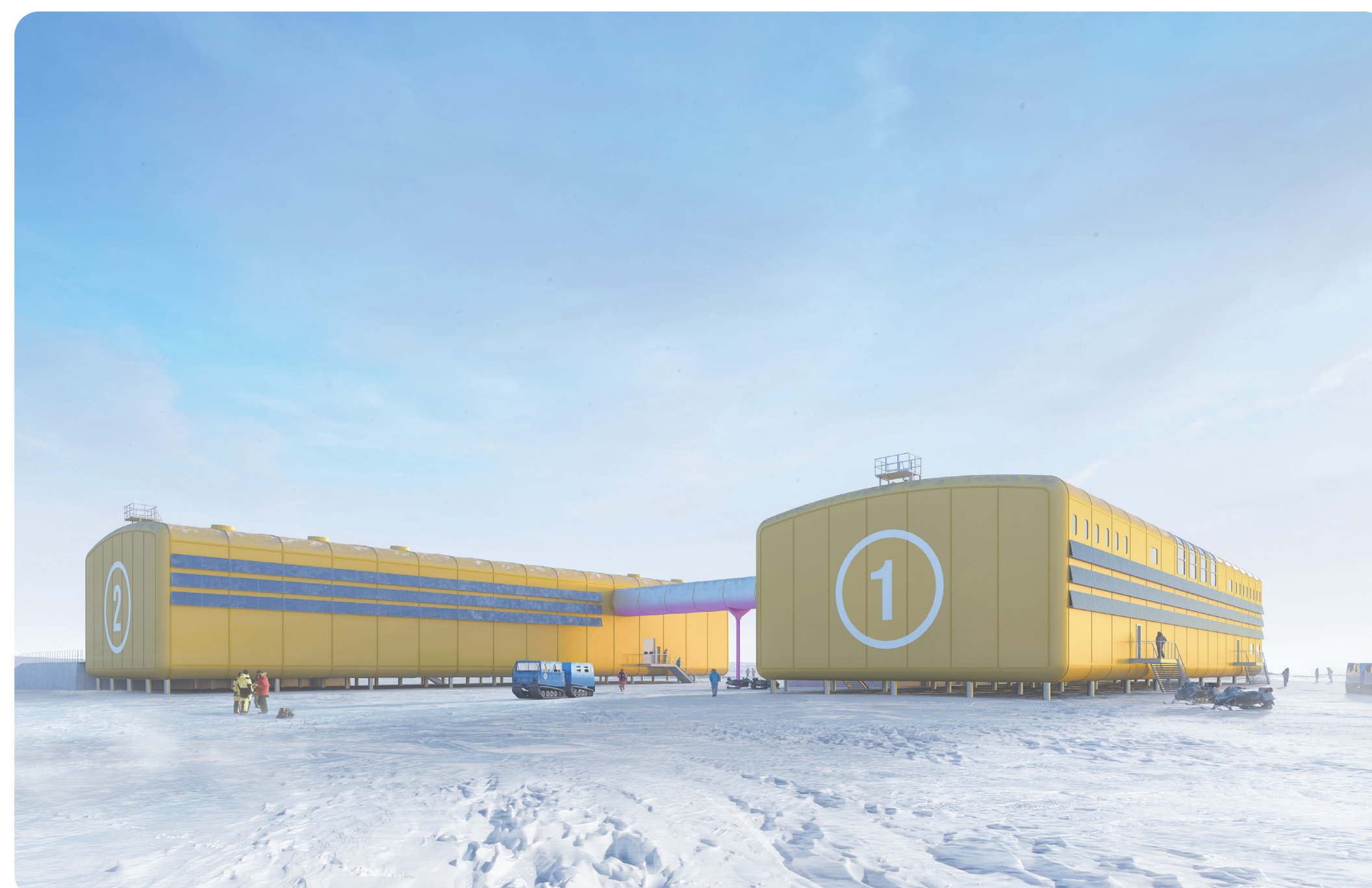
Priority infrastructure renewal at Davis Station will reduce safety risks to expeditioners and improve station operations and capability.
